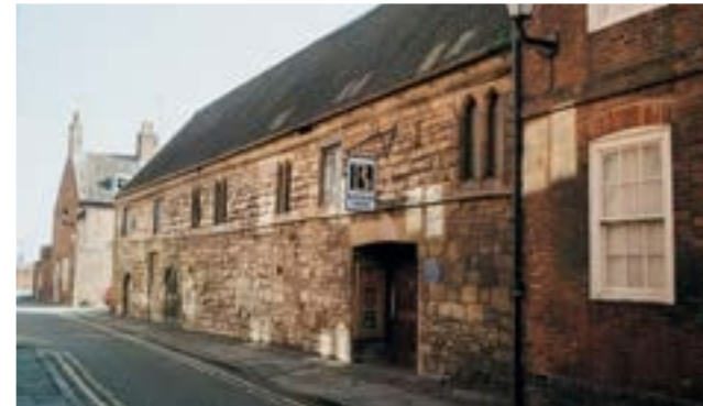
The surviving portion of the former Franciscan Friary on Spain Lane
