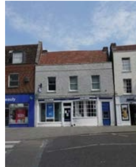
There are some bay windows at ground floor, with sash windows on upper storeys
