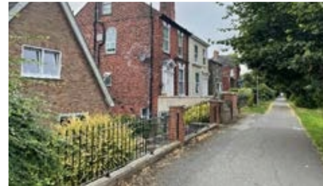
Modern alterations and infill along Witham Bank
